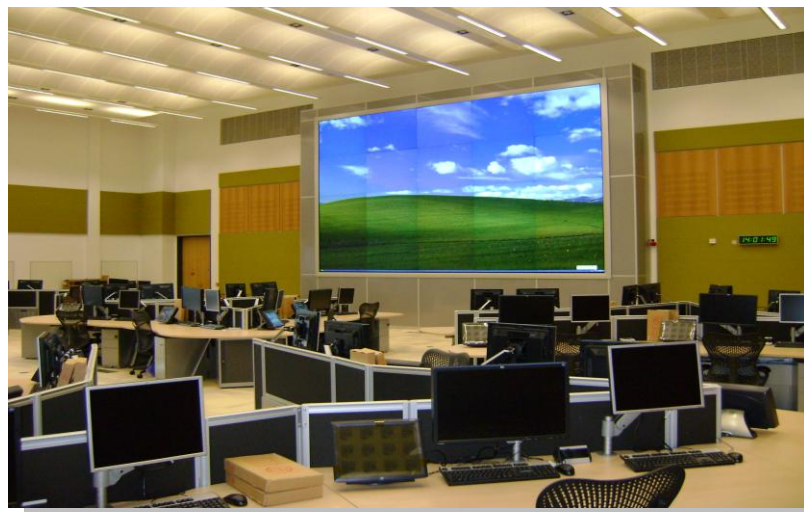
The North East RCC Control Room – contractor EADS has now placed a contract with Intergraph for the mobilising system that will be installed
